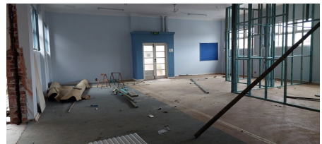
The Pemberon Visitor Centre retail space being prepared for its tenants.
