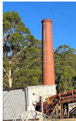
Left: Brick Chimney
